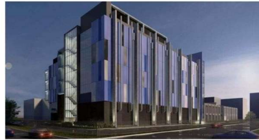
Image Credit: Macquarie Telecom Group
